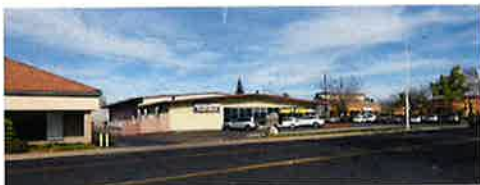
Left: View looking across East Bidwell Street towards the opportunity site.
