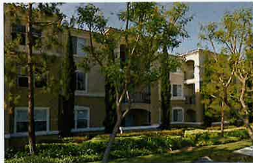
Above: Large corridor apartment building
